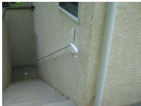
Loose Handrail
