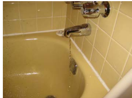
Diverter Leak
